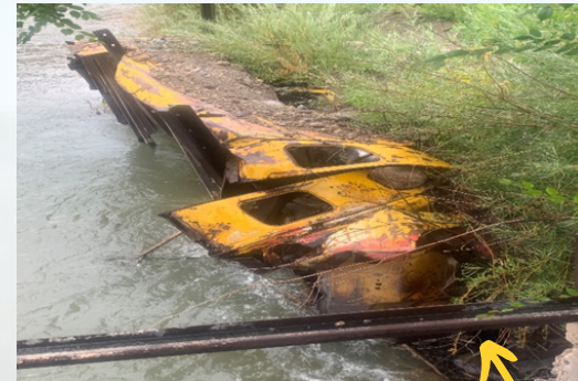
SCHOOL BUS FOR EROSION CONTROL CEDAR DITCH HEADWORKS CEDAR DITCH DIVERSION
